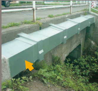
▲ Fireproof protection for optical fiber
