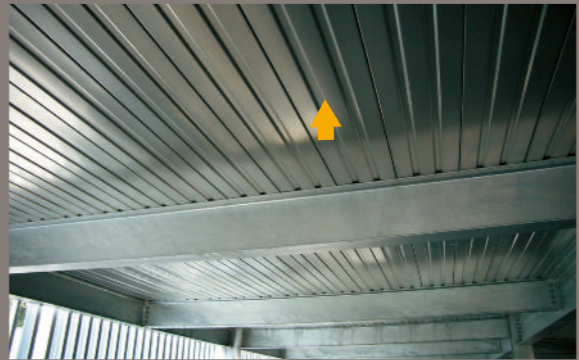
▲ Deck plate for parking lot (enlarged view)
