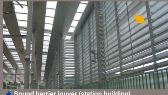
▲ Sound barrier louver (station building)
